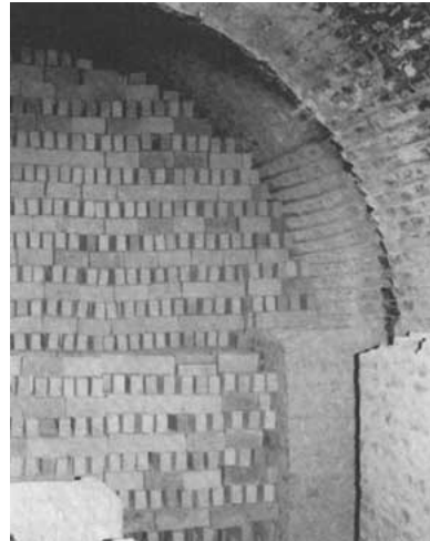
Figure VII.12 - Setting and bag walls in down-draught kiln (Ghana)
