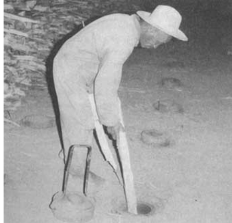
Figure VII.19 - Feeding of Hoffmann kiln with wood (Madagascar)
