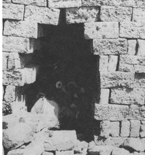
Figure VII.7 - Wood in scove tunnel (Sudan)
