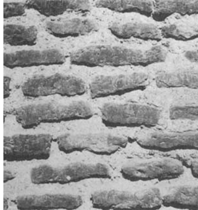
Figure VIII.3 - Old brickwork with extra-wide mortar (India)
