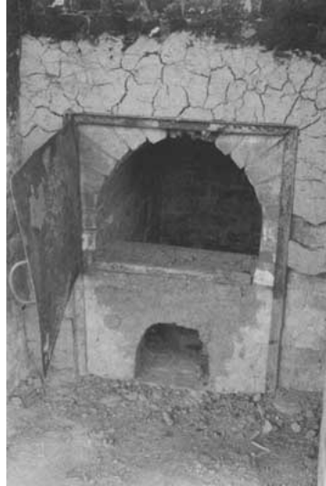
Figure VII.14 - Metal damper door for kiln grate (West Africa)
