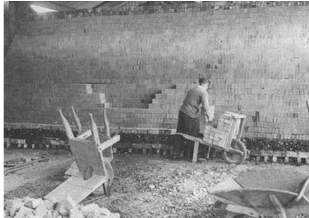
Figure VII.2 - Clamp kiln (United Kingdom)
