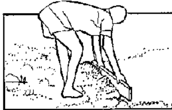
Level and smooth the kiln site.
