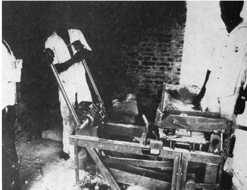
Figure IV.7. Presse Terstaram block making machine
