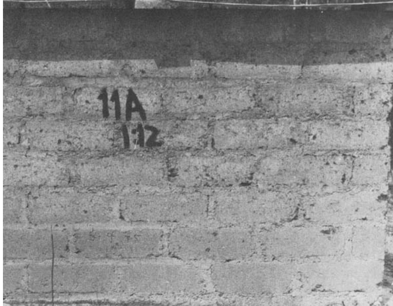
Figure I.2. Lime-stabilised soil blocks after 3 year's exposure in Ghana
