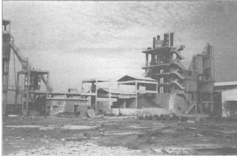
CRI- MVSK Cement plant
