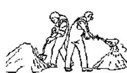
Begin mixing by turning the soil on the ground using a shovel.
