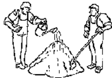
Moisten the mix using a watering can.
