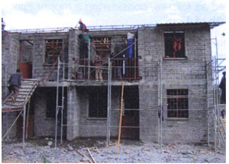
Starting the roof construction, street side view
