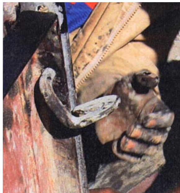
Inserting the clamp into a drill-hole of the formwork...
