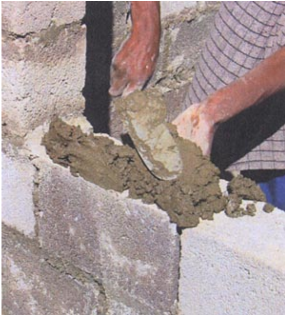
Putting the mortar on top of the last layer
