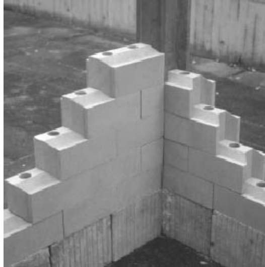
7-15 Improved interlocking system of FEB, Kassel, 2001
