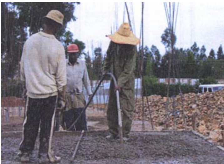
Construction of foundation using compactor
