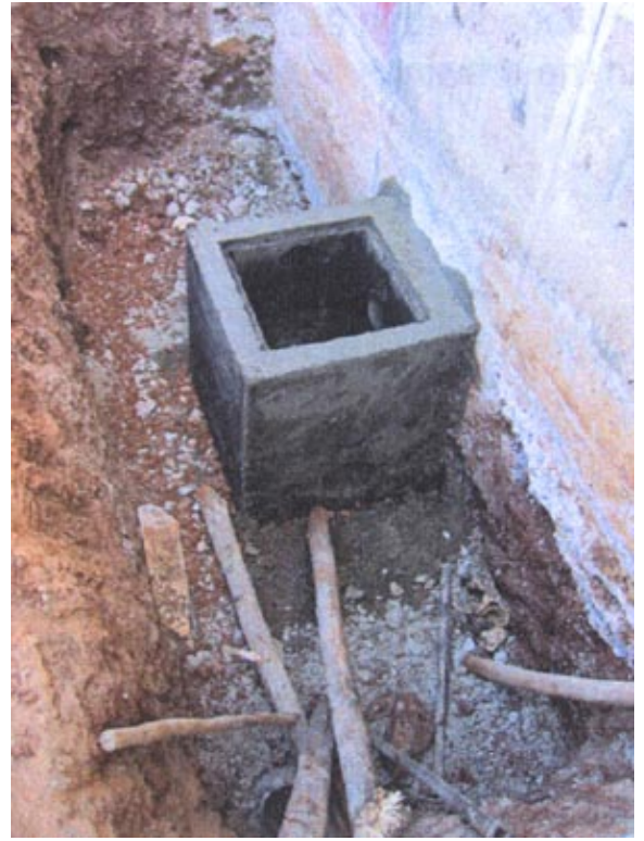
The pit for the manhole
