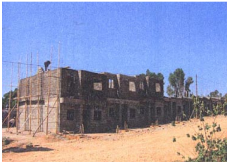
Finishing the upper floor, backyard view
