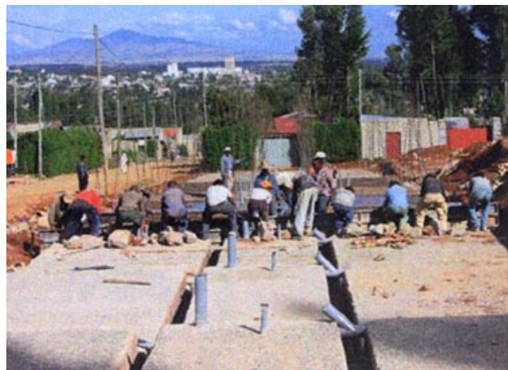
Sanitary pipes are installed
