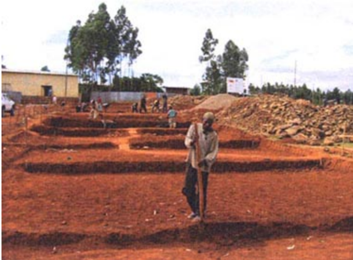
Levelling for the foundation is made
