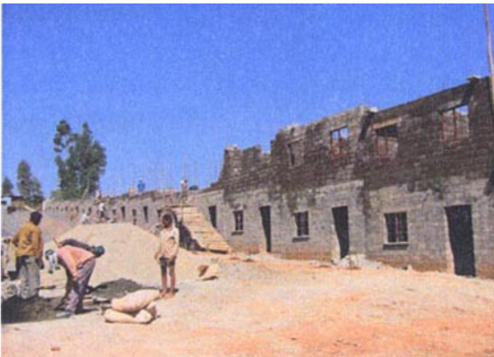
Finishing the walls of the upper floor, street side view
