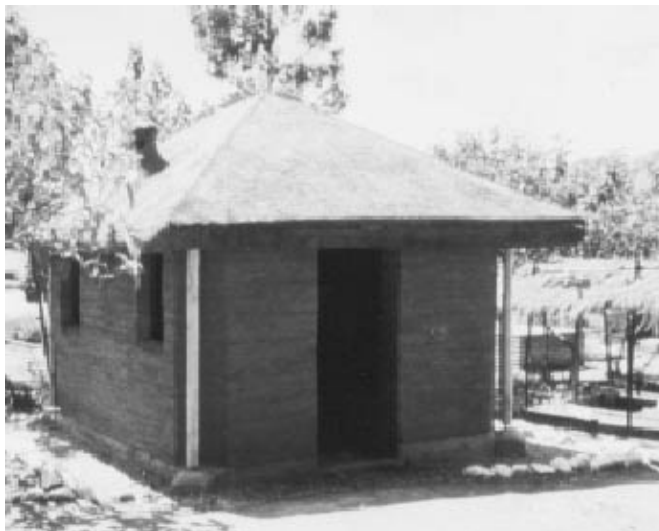
Figs. 12–5 and 12–6 show solutions of projects which were described in chapter 6.4. In the first case the columns are positioned inside, in the second case outside the walls.
