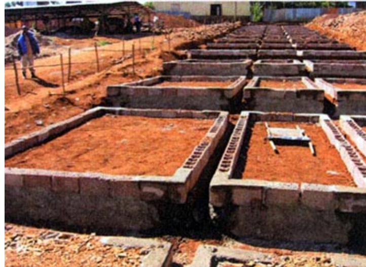
Preparation for combined strip and mat foundation
