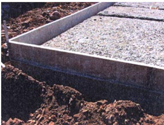
A formwork for foundation, panels mounted on top of each other, side by side and at the edge
