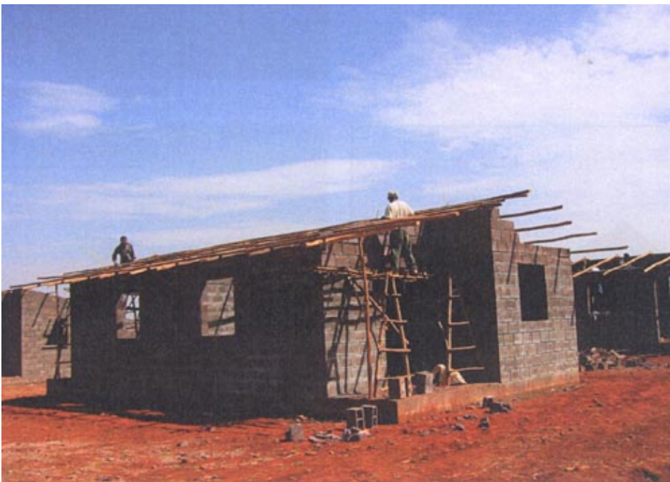
Construction of Houses in Bahir Dar
