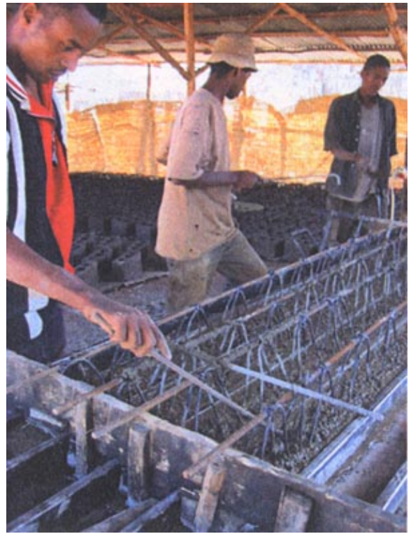
Spreading the concrete, using a bend bar
