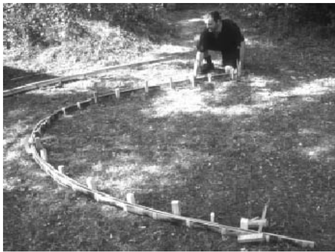
15-7 Construction of the arc with split bamboo
