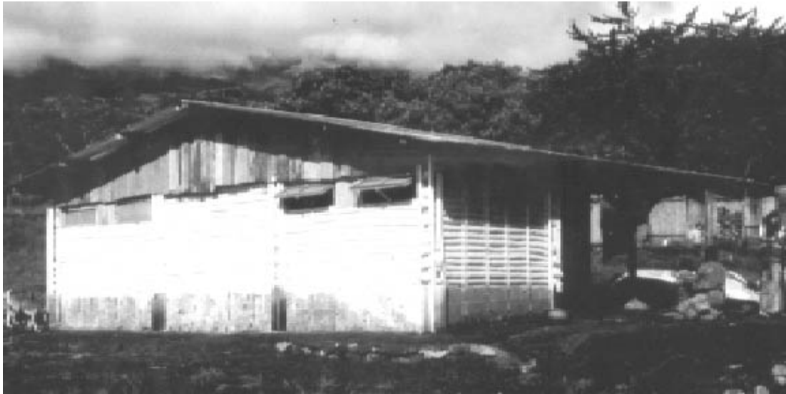
9-7 Earthquake resistant low-cost housing prototype, Guatemala 1978
