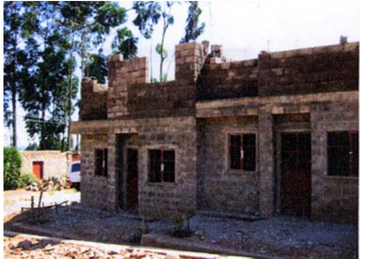
Starting the upper floor, street side view
