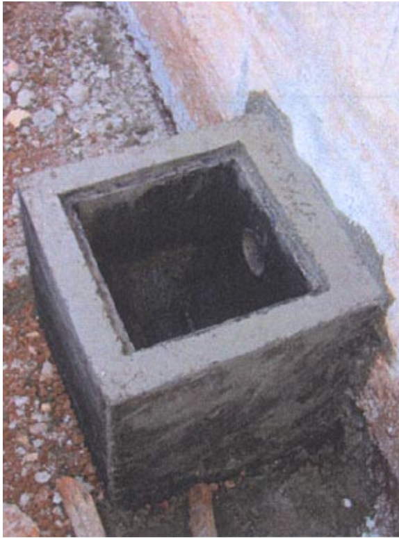
The cast manhole
