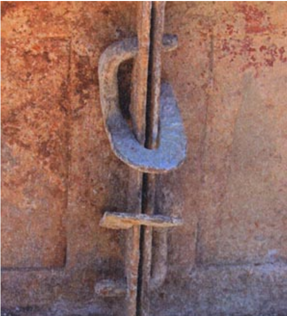
Two clamps mounted on formwork for foundation
