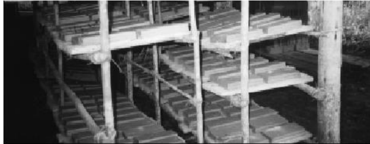
Fig. 6: Simple method of drying floor tiles on racks under a grass roof
