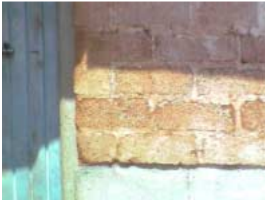
Balram block walling (self build)
