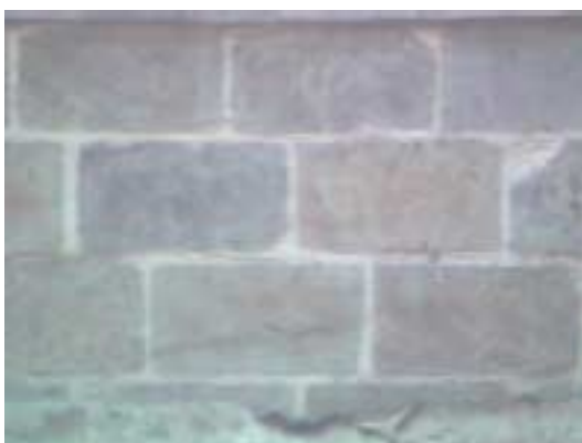
Stone cladding over bricks
