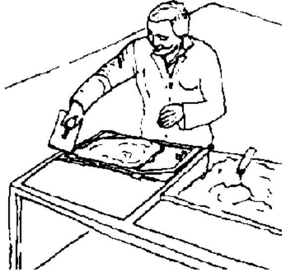
Figure 40. Screeding the mortar in the frame
