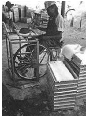
1. Placing mortar on the screeding surface
