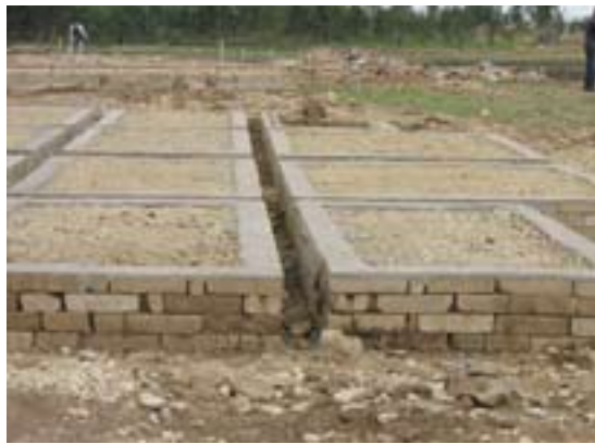
The finished foundation
