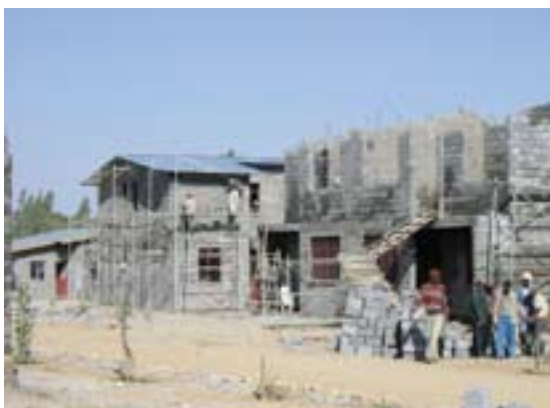
Starting first floor
