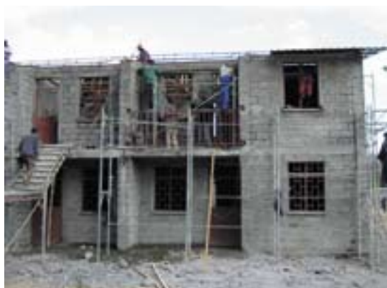
Starting the roof construction, street side view
