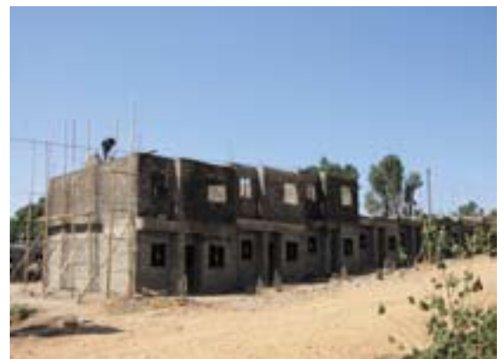
Finishing the walls of the upper floor, street side view
