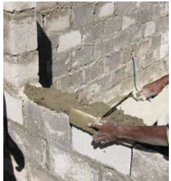
Spreading the mortar to the edge, using a piece of wood
