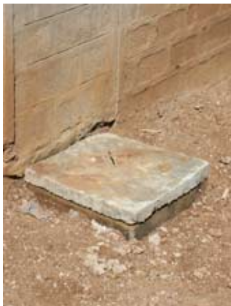
The manhole covered with a precast lid
