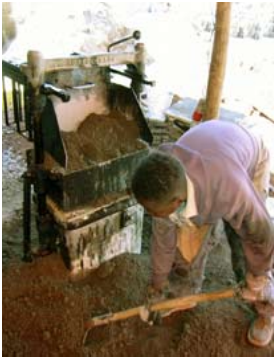
Filling in concrete while the machine is already vibrating
