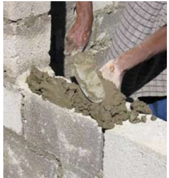
Putting the mortar on top of the last layer
