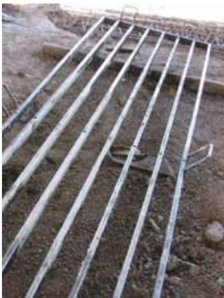
Mould for the pre-cast beams
