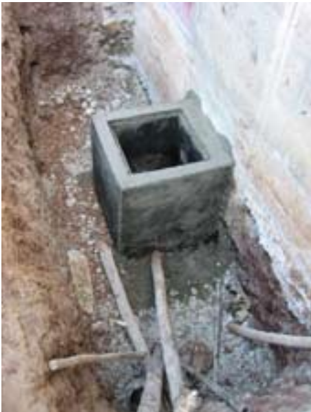
The pit for the manhole
