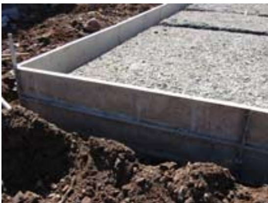
A formwork for foundation, panels mounted on top of each other, side by side and at the edge
