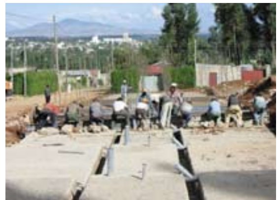
Sanitary pipes are installed
