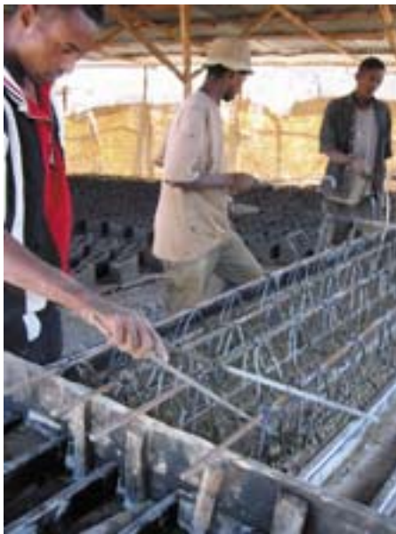
Spreading the concrete, using a bend bar
