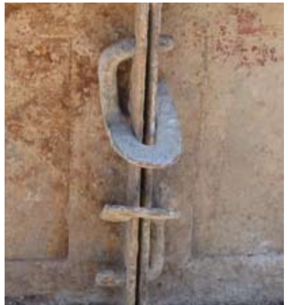
Two clamps mounted on formwork for foundation
