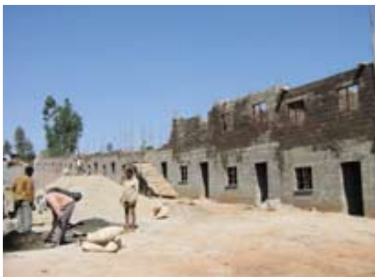
Finishing the upper floor, backyard view
