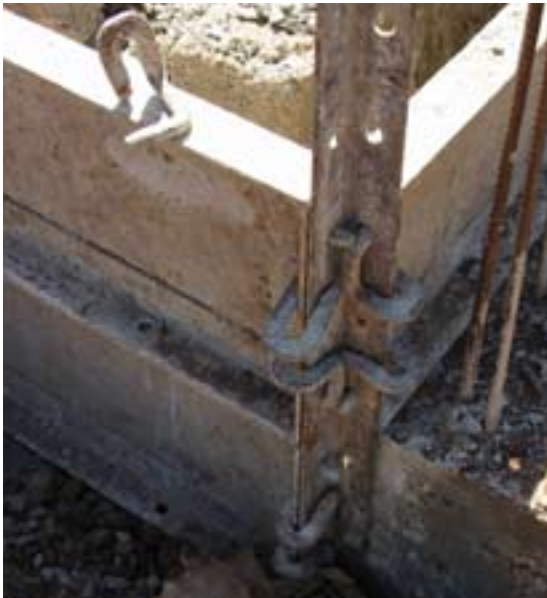
The edge of a formwork-assembly for foundation
