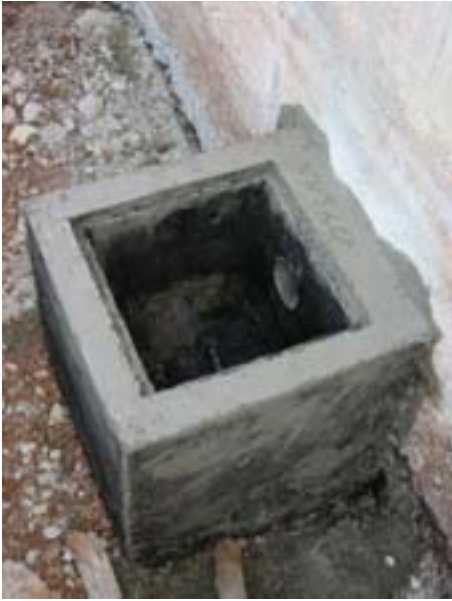
The cast manhole
