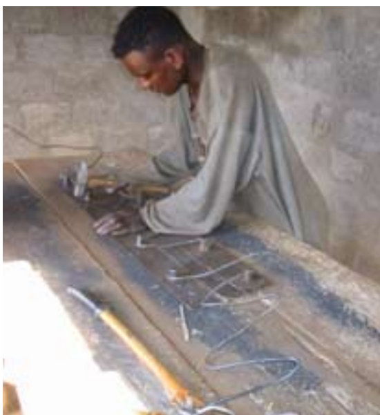
Starting the new segment
