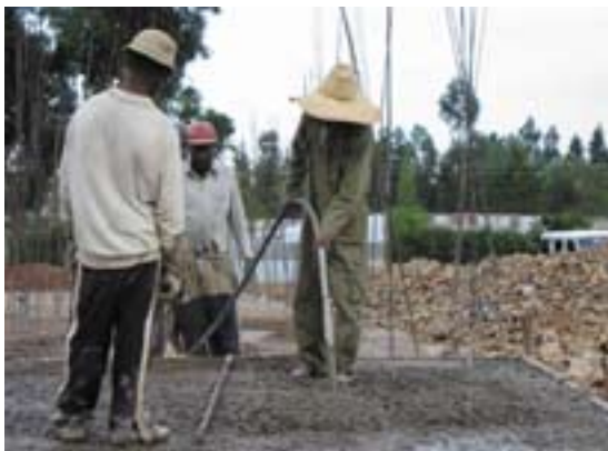
Construction of foundation using compactor
