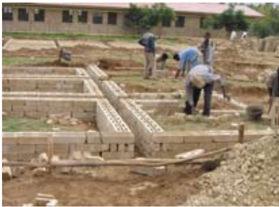
Lost formwork for foundation
