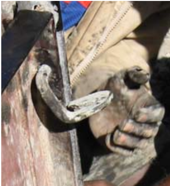
Inserting the clamp into a drill-hole of the formwork...
