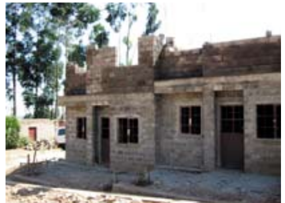
Starting the upper floor, street side view
