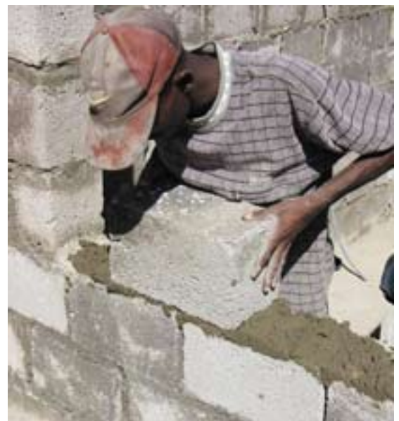
Placing the HCB with the closed bottom up
