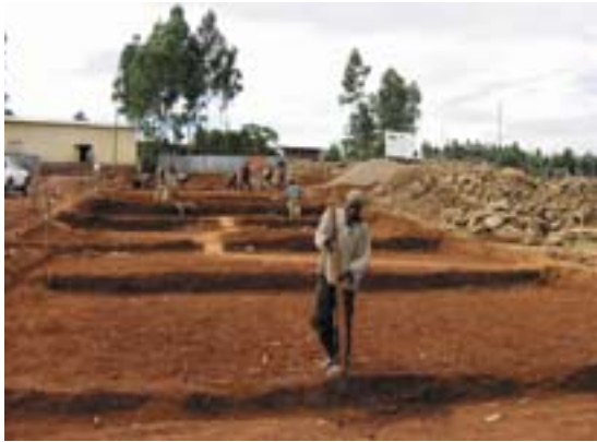
Levelling for the foundation is made
