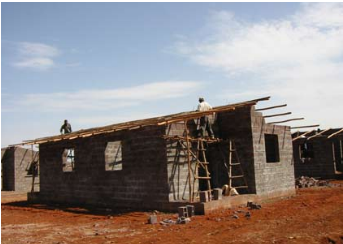
Construction of Houses in Bahir Dar
