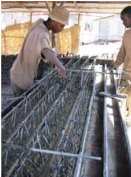
Filling in concrete by hand
