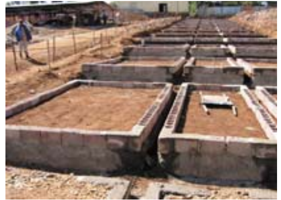
Preparation for combined strip and mat foundation
