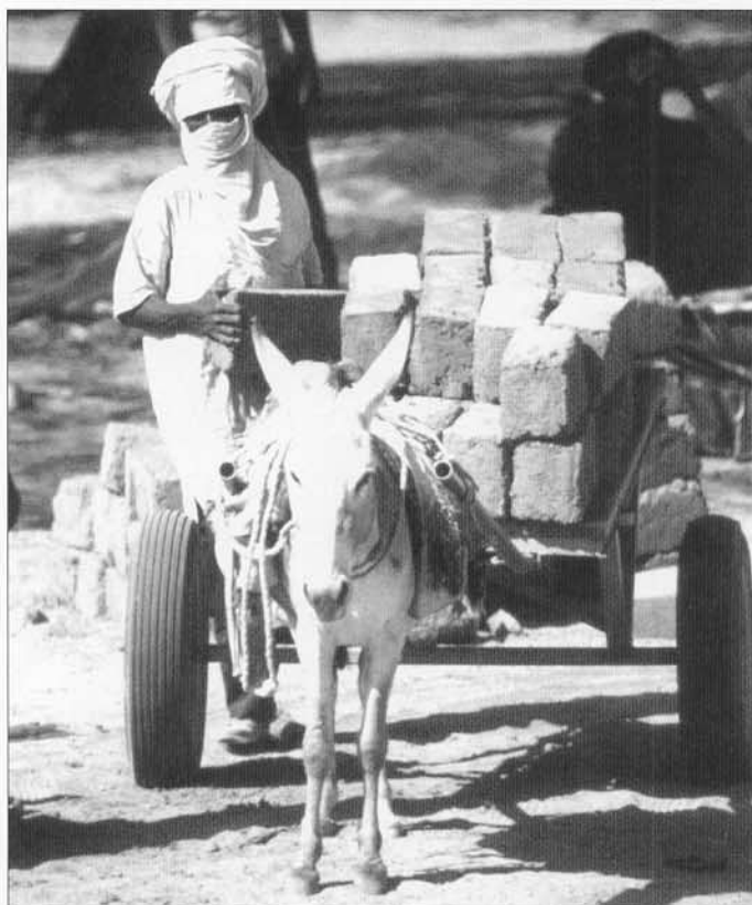
Figure 1 Bricks made using simple wooden moulds and dried in the sun
