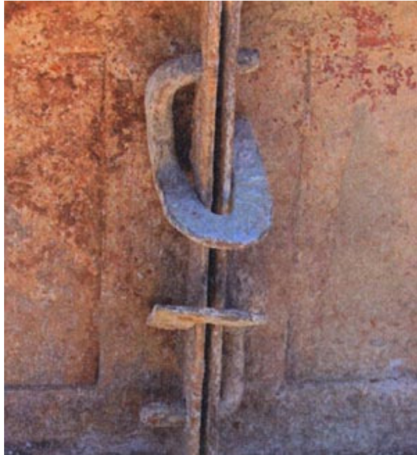
Two clamps mounted on formwork for foundation
