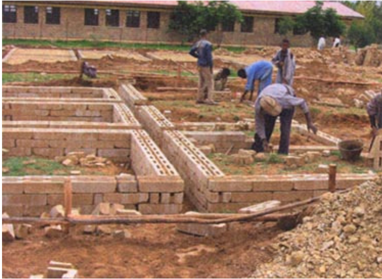
Lost formwork for foundation
