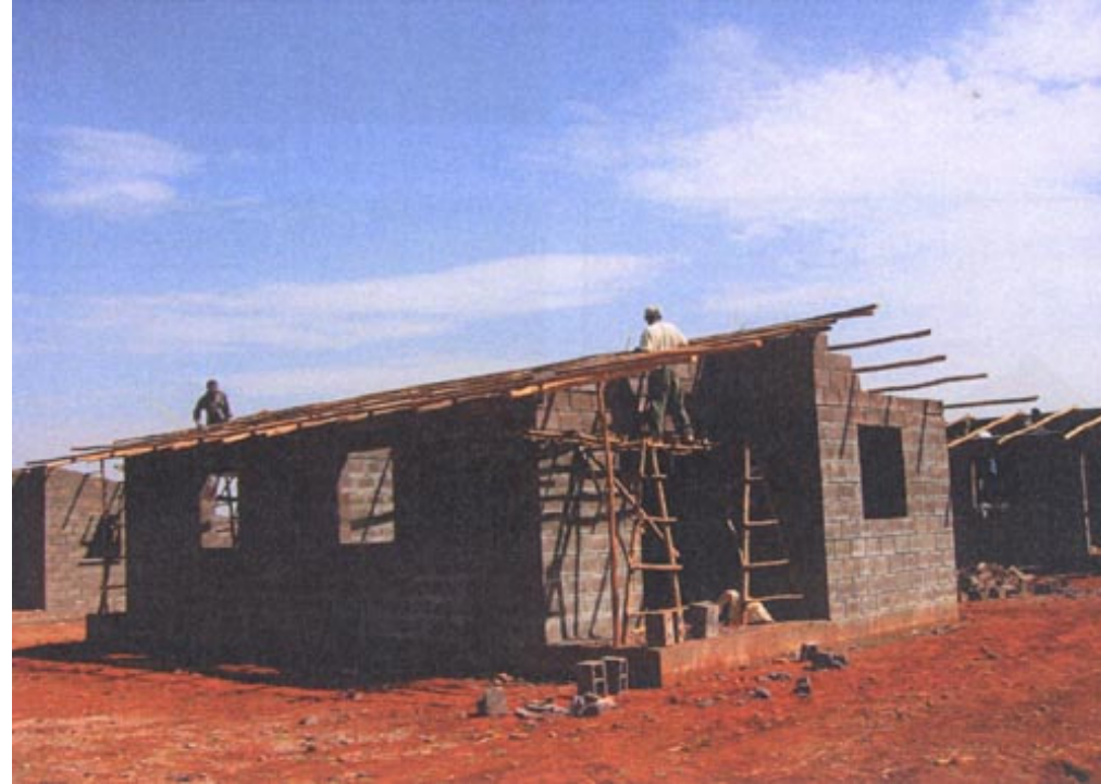
Construction of Houses in Bahir Dar
