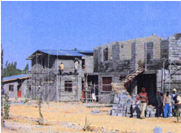
Starting first floor
