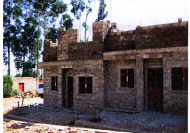
Starting the upper floor, street side view
