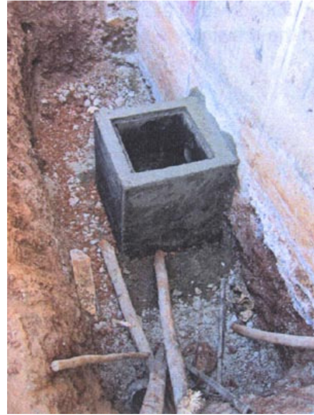
The pit for the manhole
