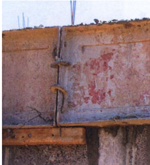
A formwork for a slab, fixed by additional wires bound to the reinforcement of the slab
