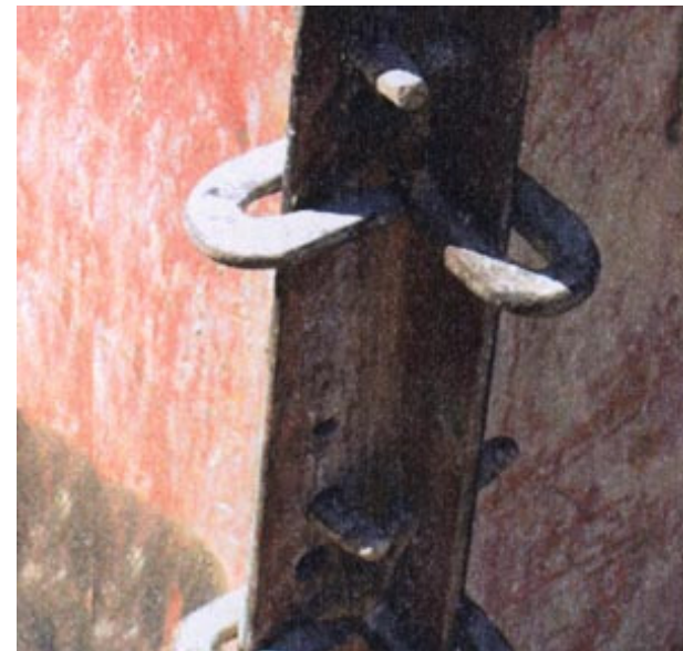
Inserting the clamp into a drill-hole of the formwork...
