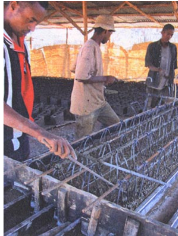
Spreading the concrete, using a bend bar
