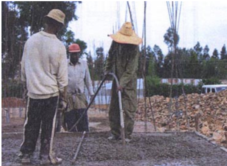
Construction of foundation using compactor
