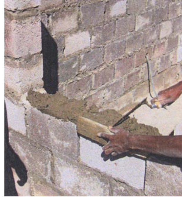
Spreading the mortar to the edge, using a piece of wood
