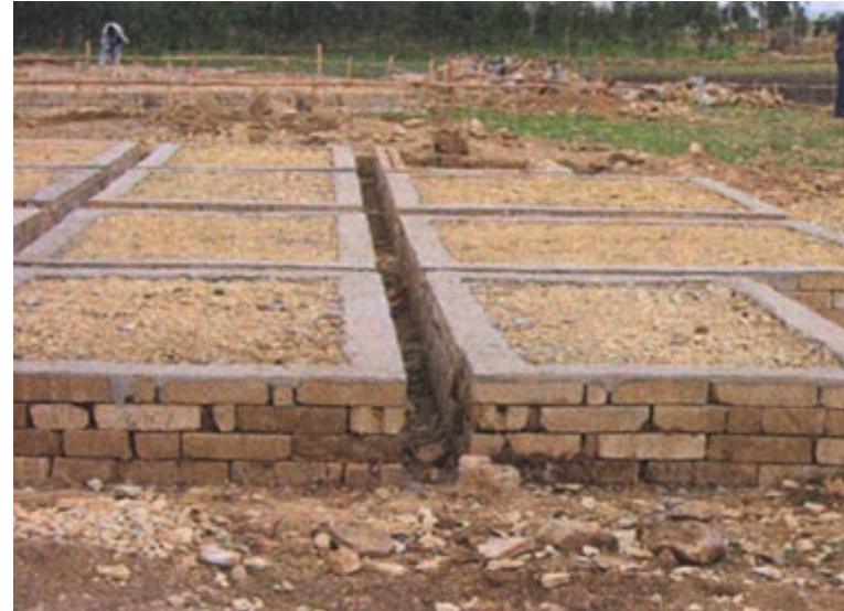
The finished foundation
