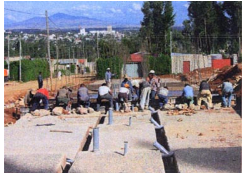
Sanitary pipes are installed
