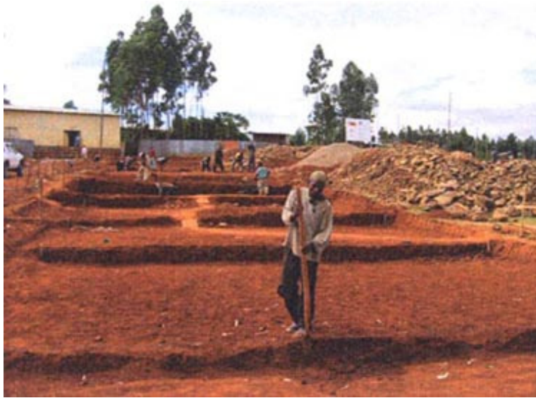
Levelling for the foundation is made
