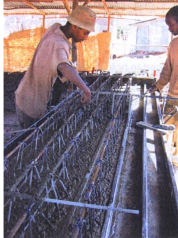
Filling in concrete by hand
