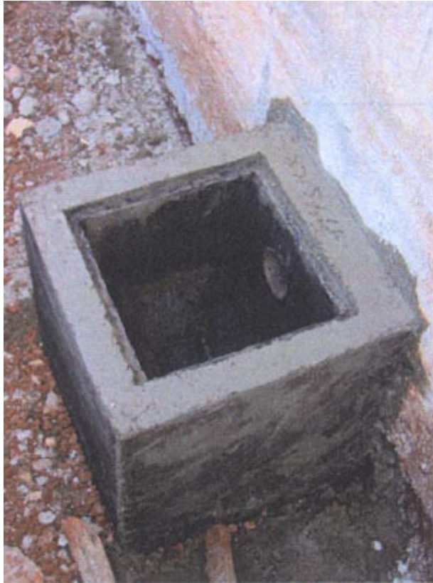
The cast manhole
