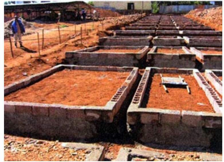
Preparation for combined strip and mat foundation
