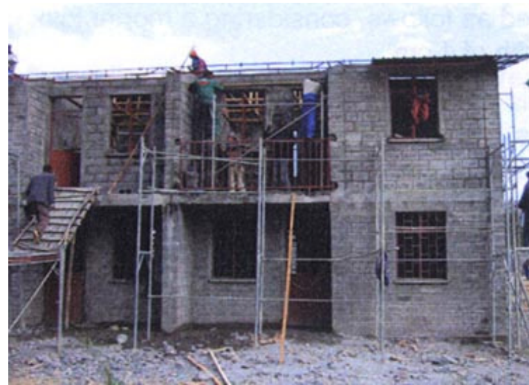
Starting the roof construction, street side view
