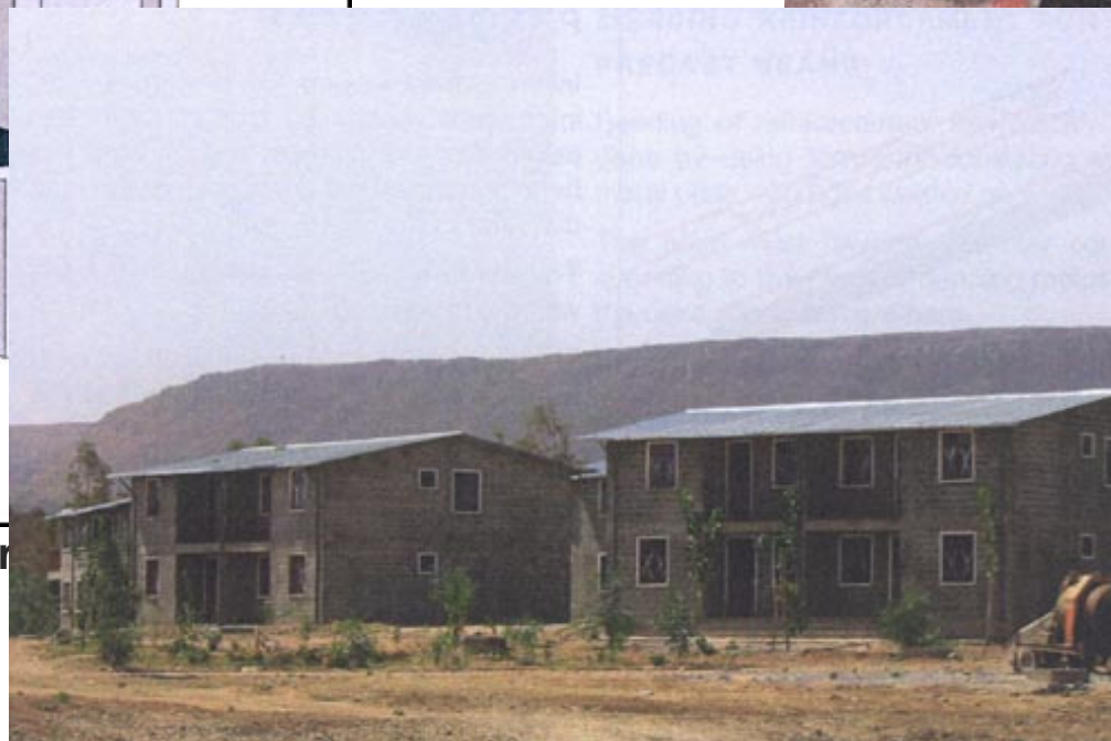
Settlement area in Mekelle
