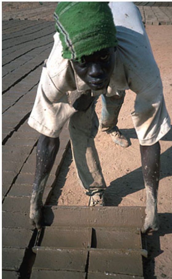
Figure 3: Brick-making using improved kiln at Kassala, Eastern Sudan. Releasing the moulds and laying bricks for drying. ©Practical Action / Mohammed Majzoub
