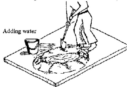
**Figure 24: Hand-mixing system**
