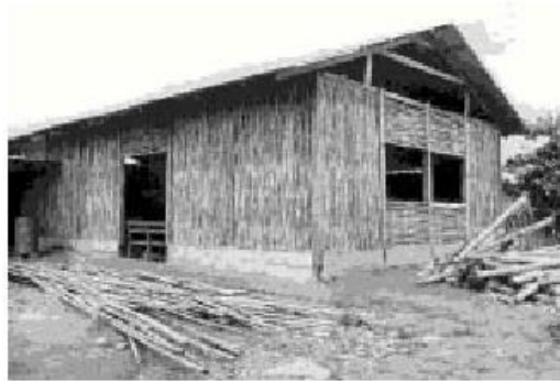
Figure 10: The Community building in Soritor during construction ITDG/Rumi Velacllaga
