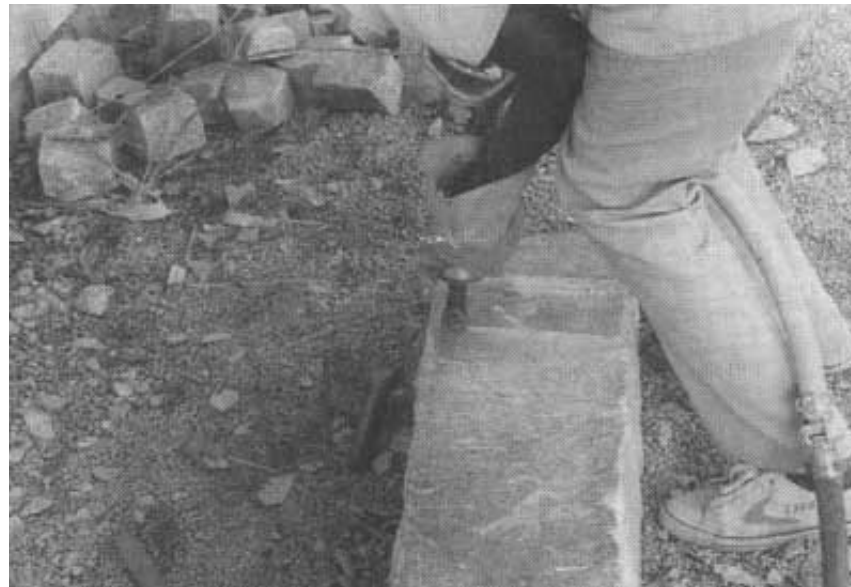
Channelling using a pneumatic hammer drill.
