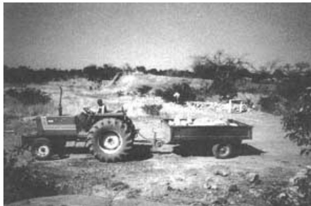
Edging curbstones being transported by tractor and trailer.
