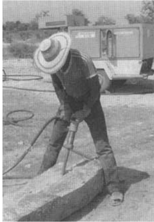
Enlarging the base of the hole.
