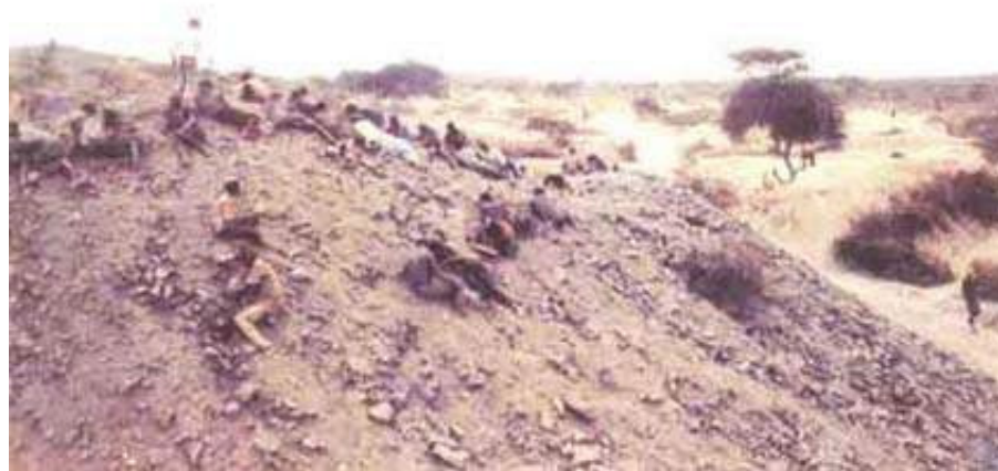
Figure 14: A Mound of Stockpiled Rock from Artisanal Mining Activities at Merelani
