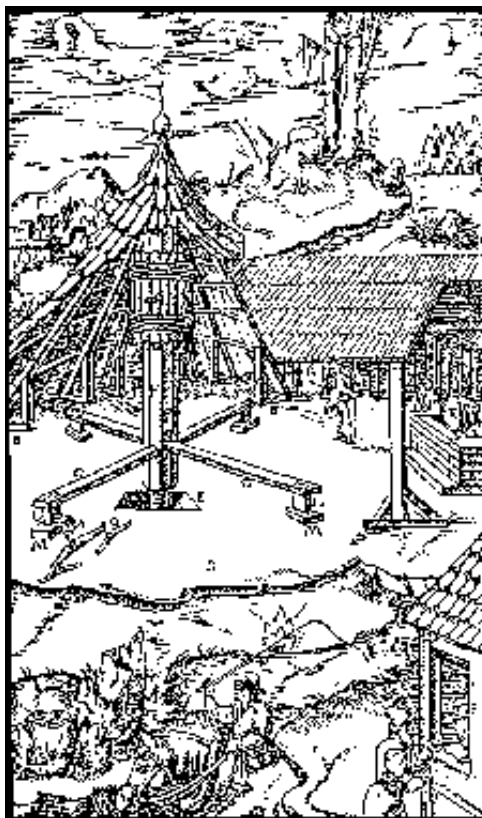
Fig.: Horse-powered whim for shaft haulage. Source: Agricola.
