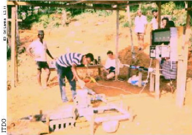
Installation of hydro system in Sri Lanka
