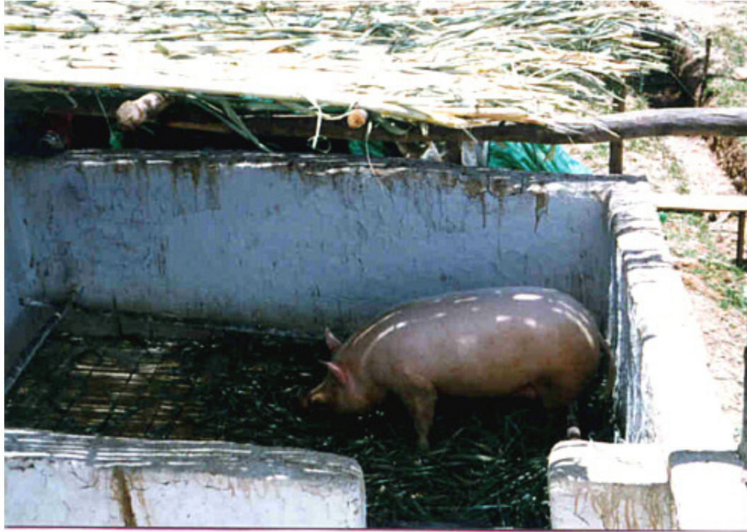
Fig. 7.2.1. An adobe pen, shaded by reeds, is an economical structure in which to raise a sow in the backyard (South America).
