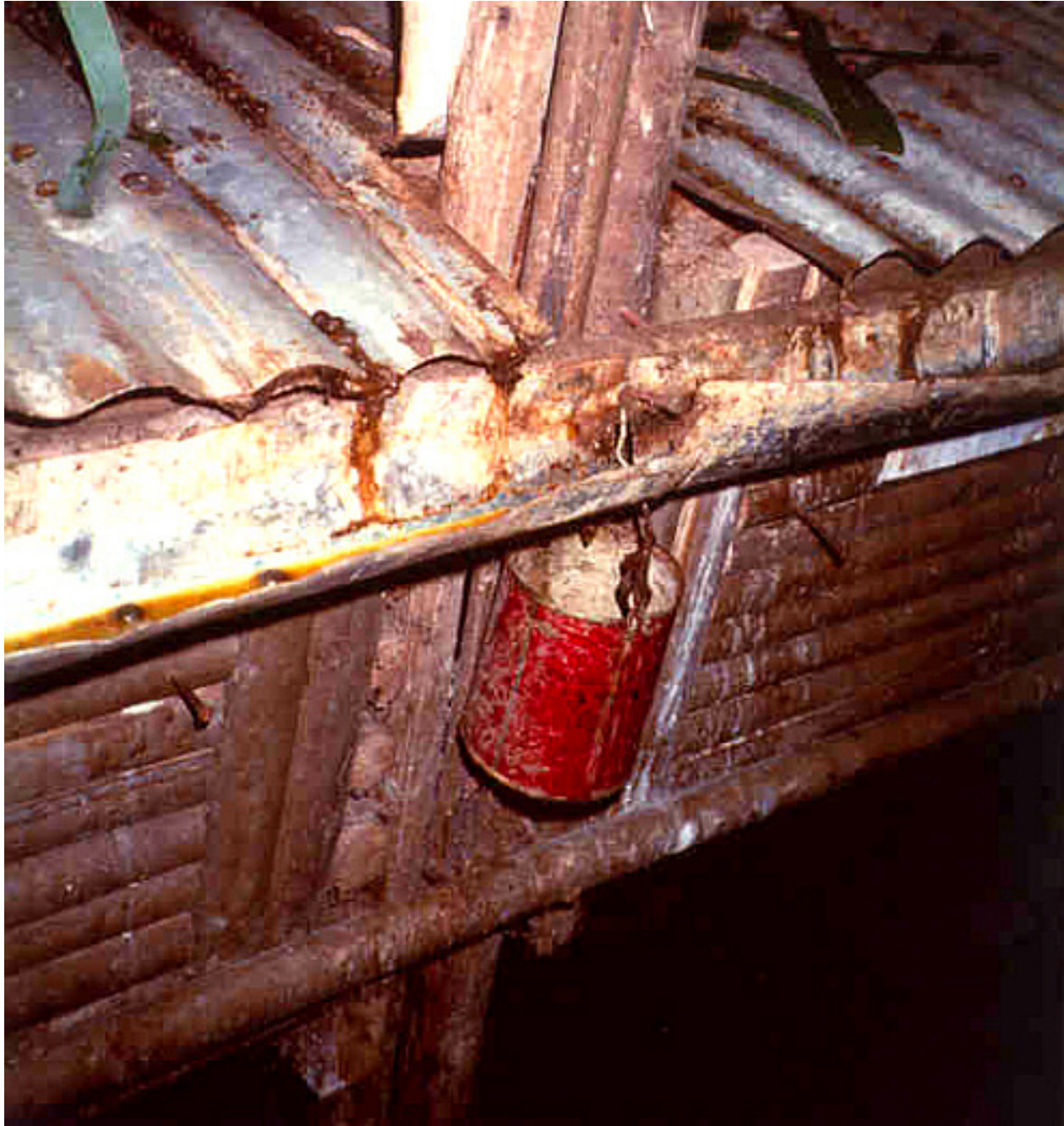
Fig. 7.2.1.22. Looking to this two-level battery
