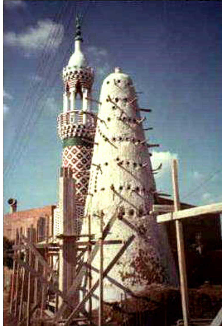
Fig. 7.1.3.5. An impressive tower to shelter pigeons. A typical scene in the Nile Delta. The tower can be compared with the minaret. Notice the analogy in the shape of the religious and utilitarian building.
