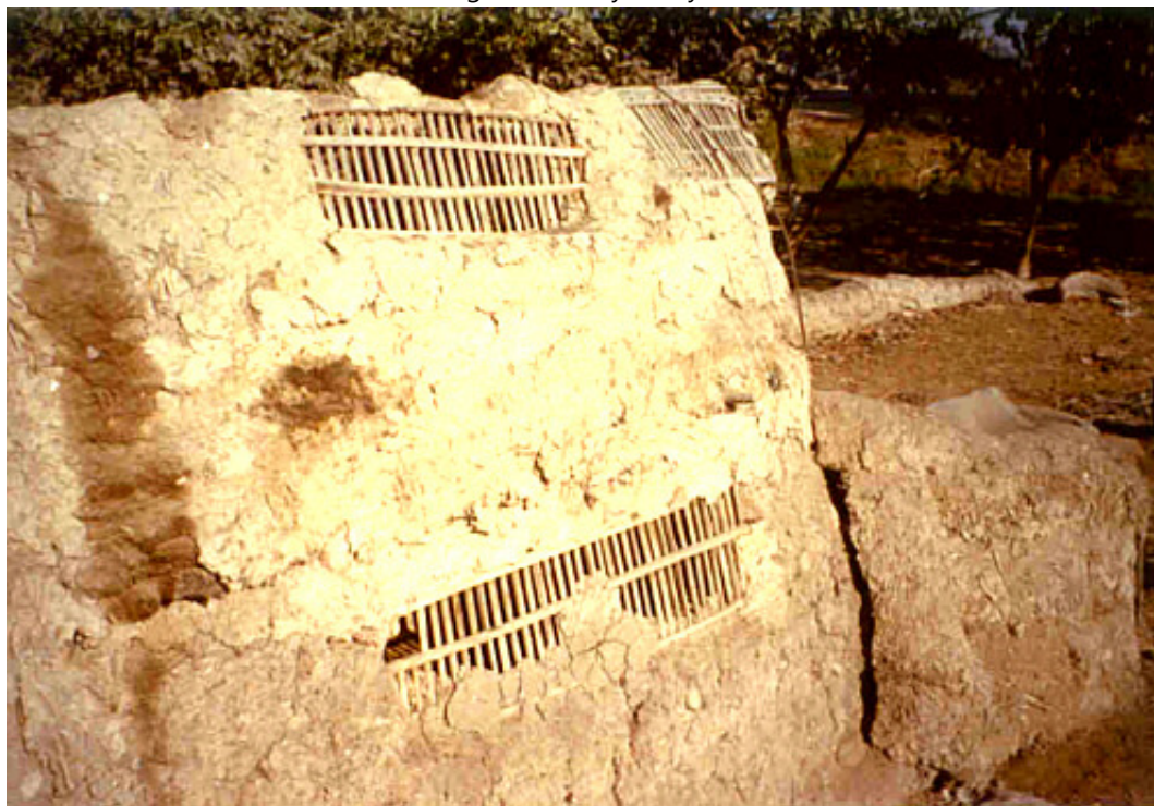
Fig. 7.1.1.10 Two superimposed mud shelters for chickens. They are cheap and efficient. The grilles to give air to the animals are made from sticks of palm leaf stems (North Africa).
