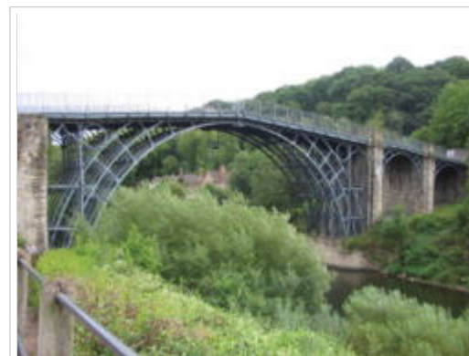
The Iron Bridge (1781) The first large bridge made of cast iron
