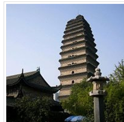
Small Wild Goose Pagoda, built by 709, was adjacent to the Dajianfu Temple in Chang'an, where Buddhist monks from India and elsewhere gathered to translate Sanskrit texts into Chinese
