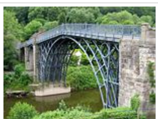
The Iron Bridge
