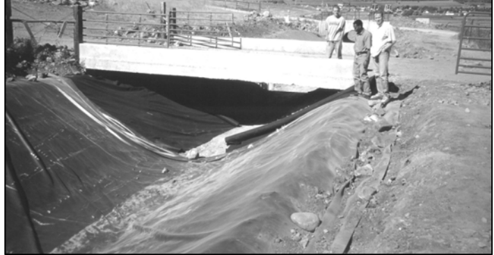
Installing plastic canal lining (courtesy R.W. Hill)
