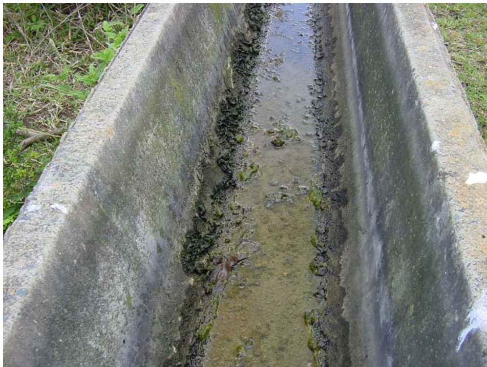
Cross section of a pre-cast concrete flume used in several irrigation systems in the Dominican Republic
