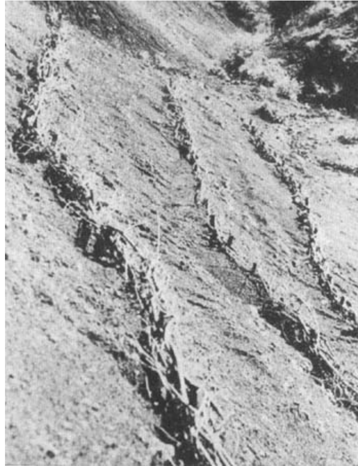
Slope protection with fascines
