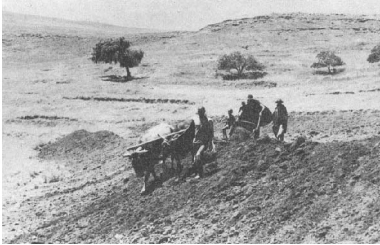
Construction of a terrace at one go (Lesotho)
