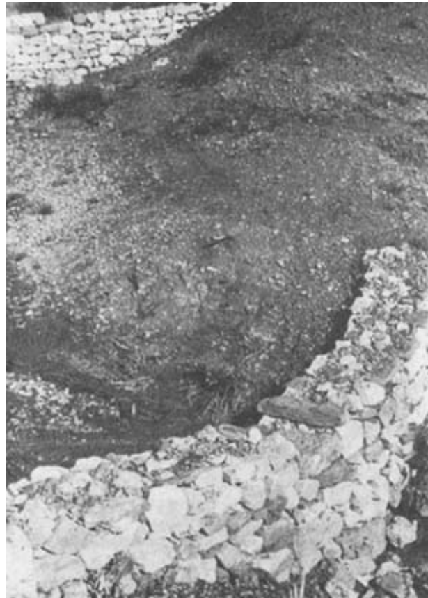
Example of a dry - stone weir
