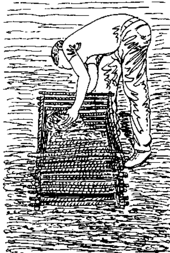
Figure 28. The frame is plastered with mud and cow-dung.
