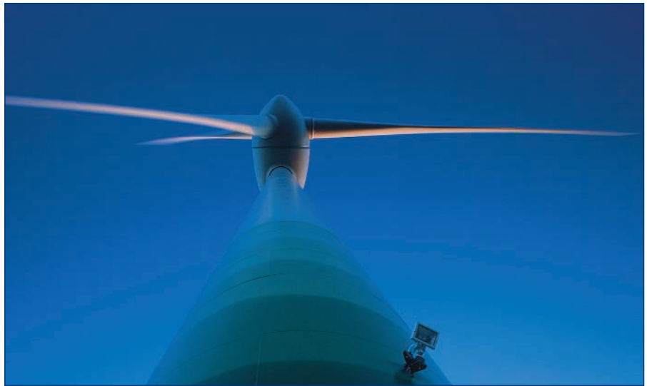
Figure 3: Close up of an Enercon wind turbine. The Green coating fades towards the middle of the tower, so that the bottom matches the green of the countryside, while the top matches the sky. (Photo courtesy of Enercon)
