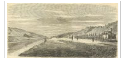
Construction of the canal
