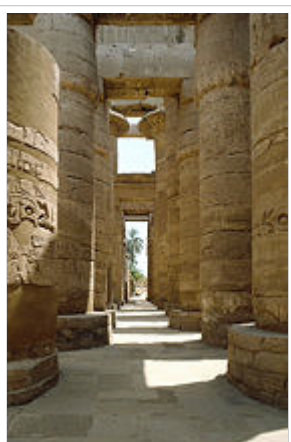
Karnak temple's hypostyle halls are constructed with rows of thick columns supporting the roof beams.
