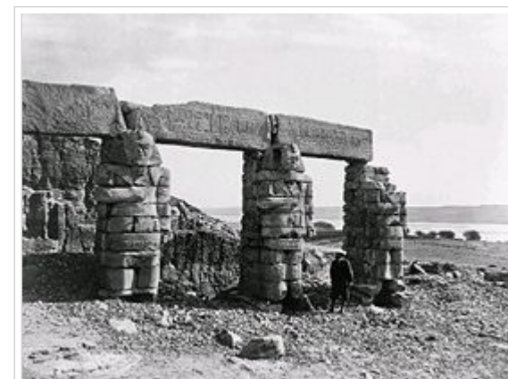
Photo of the free standing part of Gerf Hussein temple, originally in Nubia
