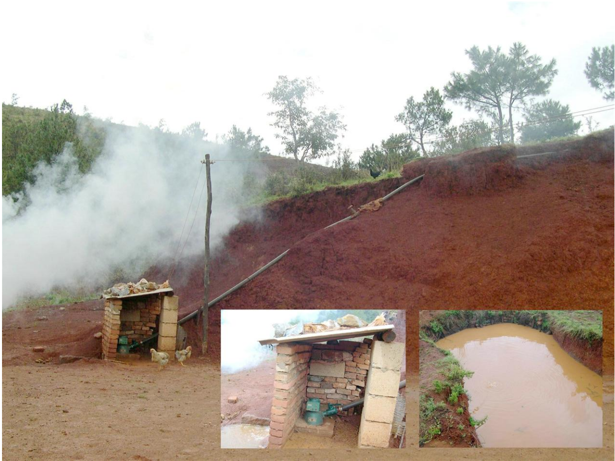
A inclined micro hydro turbine installed in the rural district.
