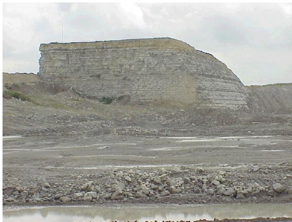
Figure 4.2: Limestone quarry formation, showing the 45° ripping technique (Copyright Halliburton Energy Services).
