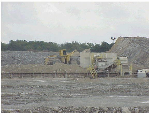
Figure 4.3: Mobile crusher and XRF unit (Copyright Halliburton Energy Services).
