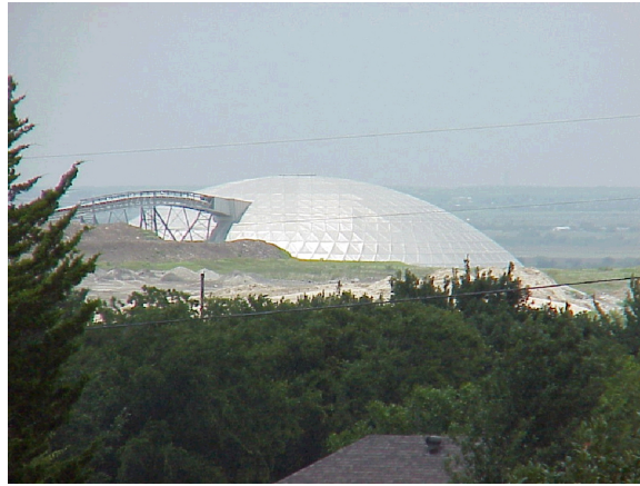
Figure 4.5: Exterior view of dome storage unit with conveyor loading port (Copyright Halliburton Energy Services).
