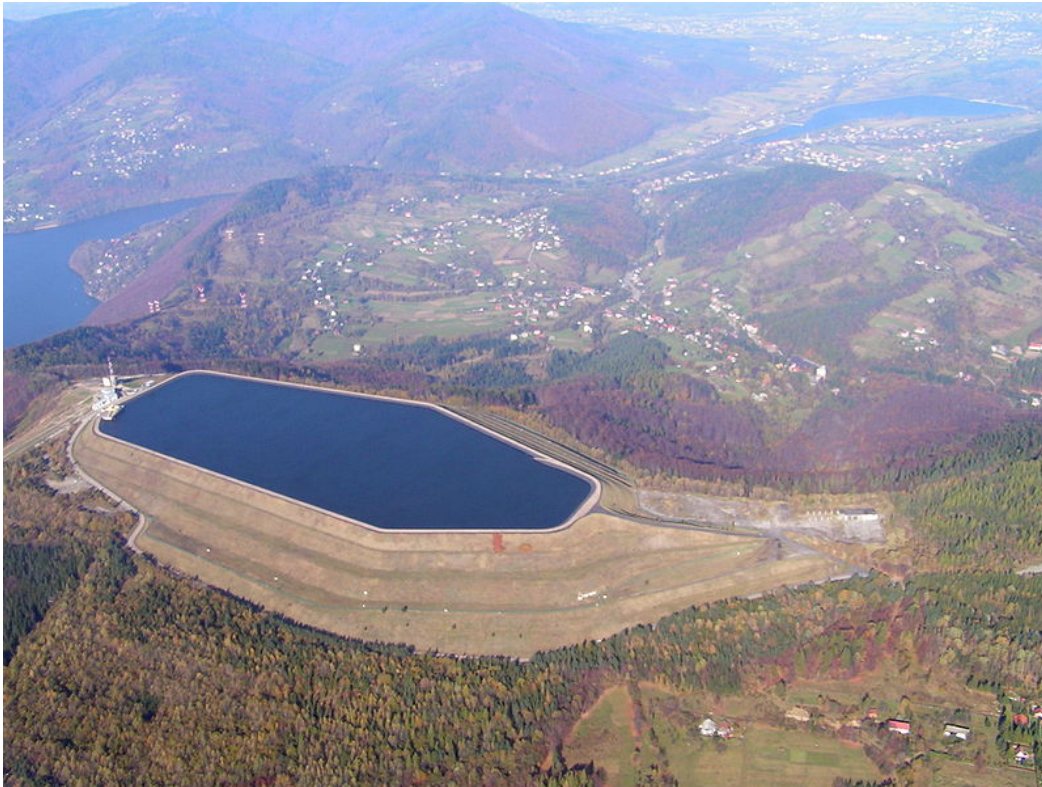
Figure 8.25: Pumped Hydroelectric Storage Upper storage reservoir for pumped hydroelectric storage, an established technology for storing large amounts of grid electricity. Source: Ongrys via Wikimedia Commons 86
