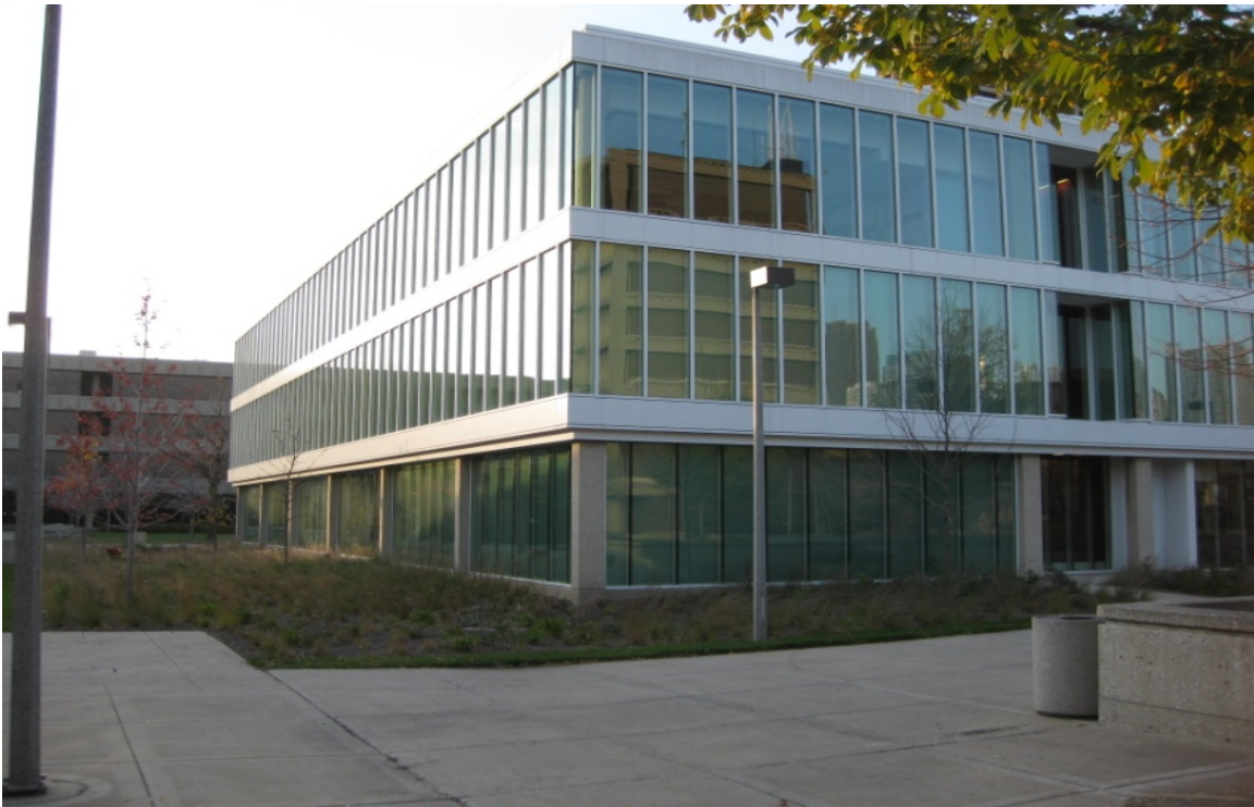
Figure 8.62: Lincoln Hall, LEED Gold Certified, University of Illinois at Chicago Lincoln Hall, LEED Gold certified building on the University of Illinois at Chicago campus. Features include geothermal heating and cooling, solar photovoltaic rooftop system, low-emittance, high-U windows, day-lighting, native planting, bioswales for stormwater management, and use of recycled materials. Source: UIC Office of Sustainability 177
