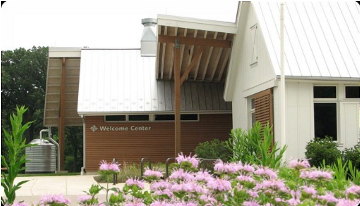
Figure 11.7: A Rain Barrel Collection System This "green" building (Ryerson Woods Welcome Center, Lake County (Illinois) Forest Preserve District) uses both a rain barrel to collect stormwater draining from the roof, and a rain garden to help infiltrate precipitation. Source: Jaffe, M., et al. (2010) (p. 542), Fig. 12, p. 116.
