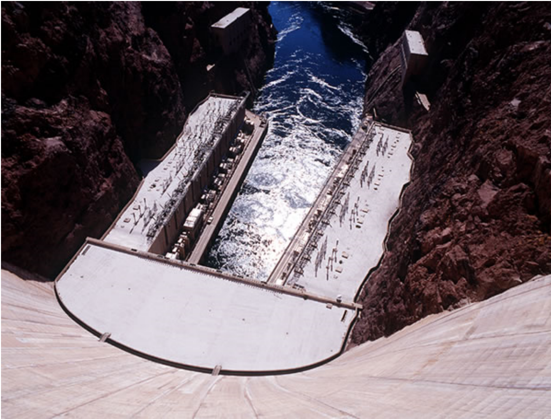
Figure 8.13: Hoover Power Plant View of Hoover Power Plant in Colorado as seen from above. Source: U.S. Department of the Interior 42
