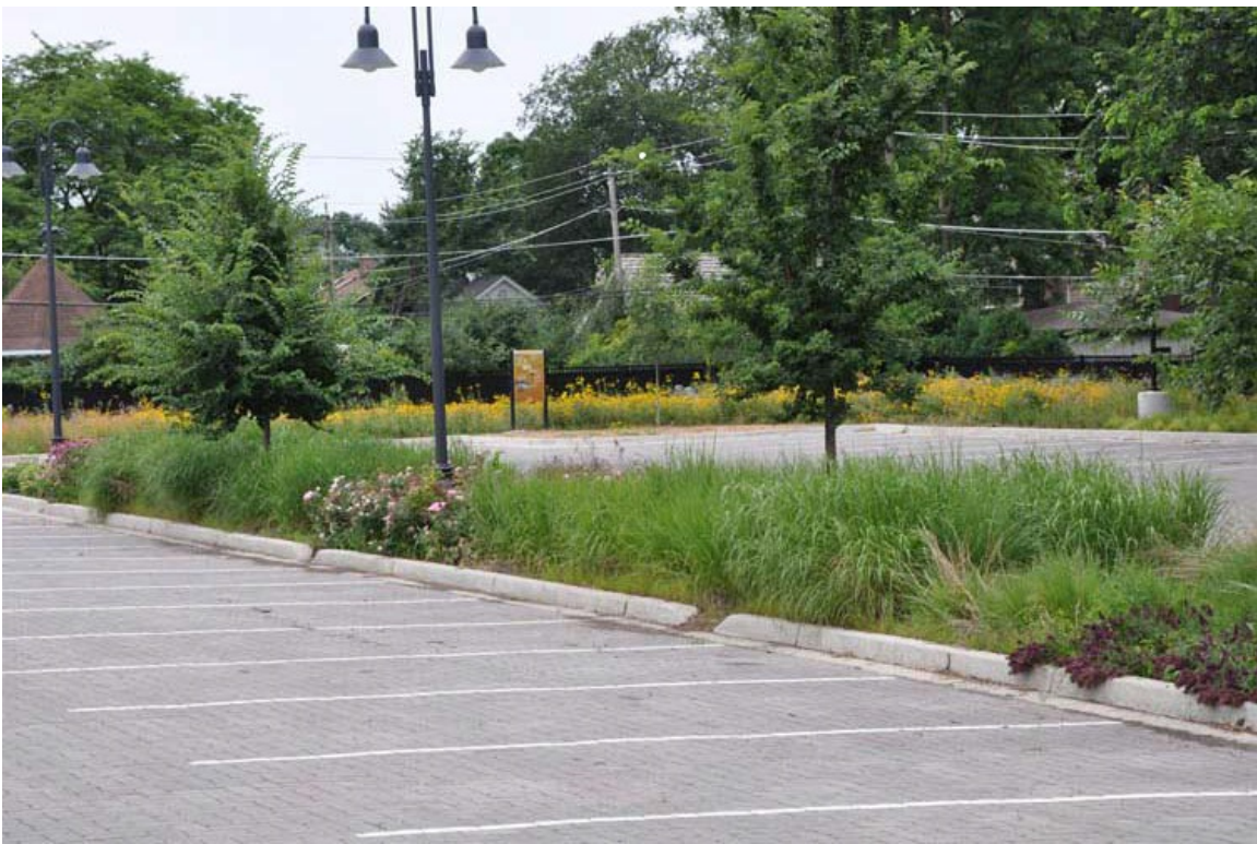
Figure 11.6: Permeable Paving & Vegetated Swales Permeable paving drains into a vegetated swale as part of Elmhurst College's (in Illinois) parking lot's "green" stormwater management system. Source: Jaffe, M., et al. (2010) (p. 542), Fig. 14, p. 117.
