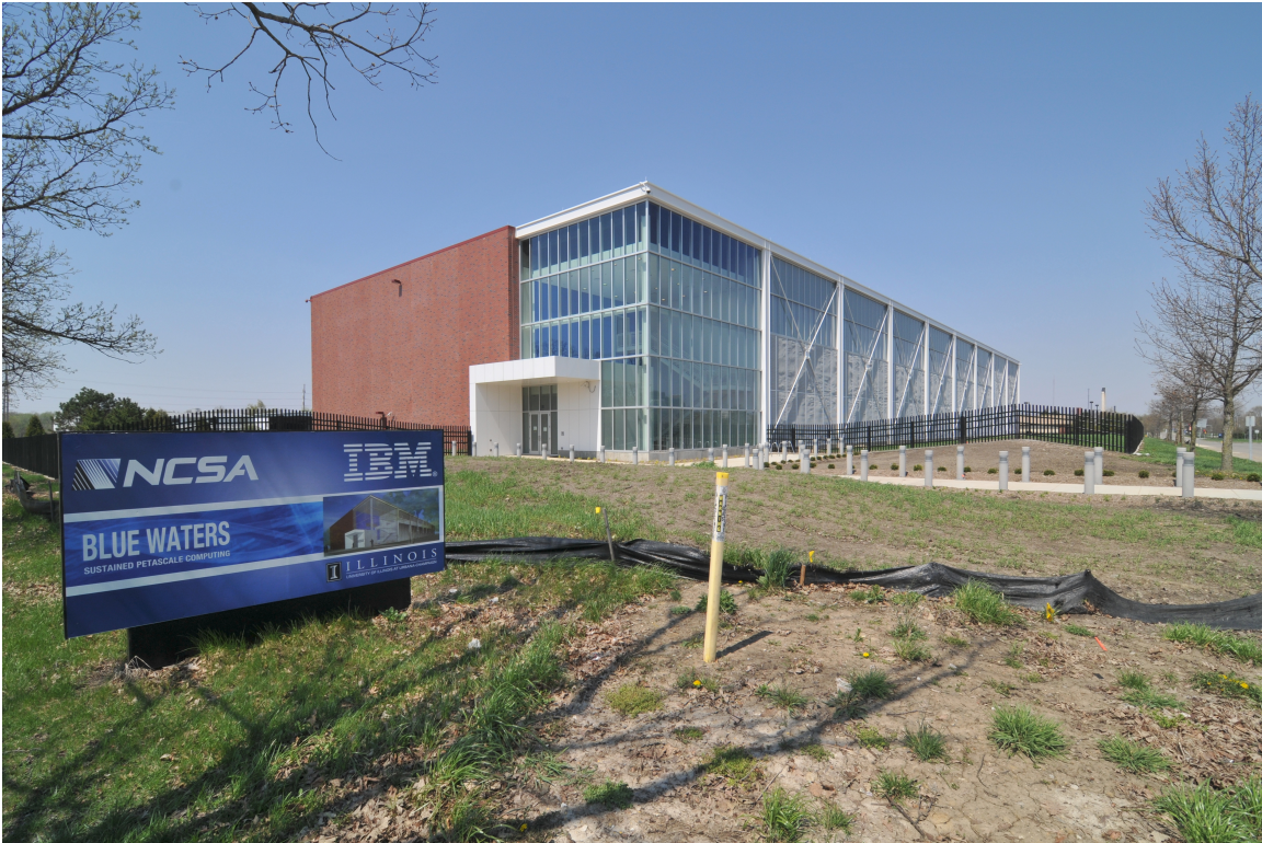
Figure 3.43: Petascale Computing Facility The petascale computing facility “Blue Waters” located at the University of Illinois at Urbana-Champaign. Source: HorsePunchKid via Wikimedia Commons 58
