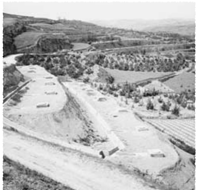
When it is raining, the ditches can lead water collected from the road and hill slope to the two rows of tanks. The tank water is used to irrigate crops and trees on the lands below. At the right below, land is sheeted with plastic films to prevent erosion and raise soil temperature. Photo: Author.
