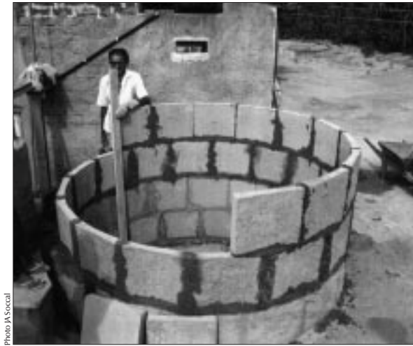
A plate cistern being built in Pedra Lavrada county, Paraíba, Brazil.
