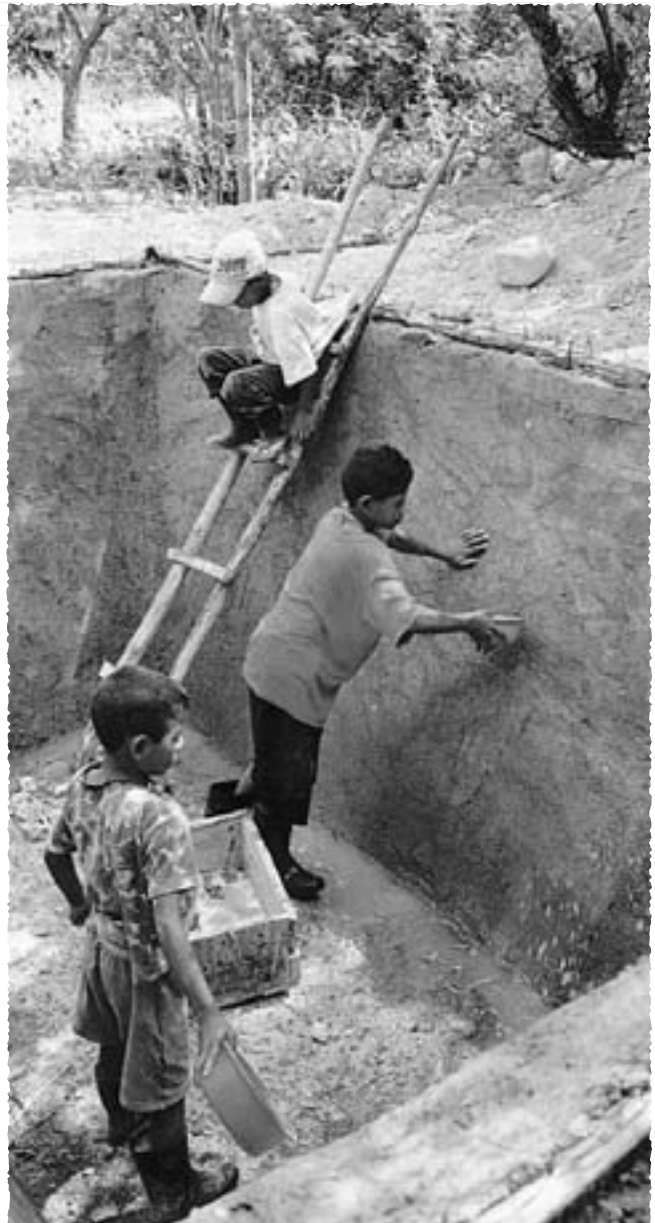
Lining the microtank, Sabannah Grande. Photo: Anita Ingevall.
