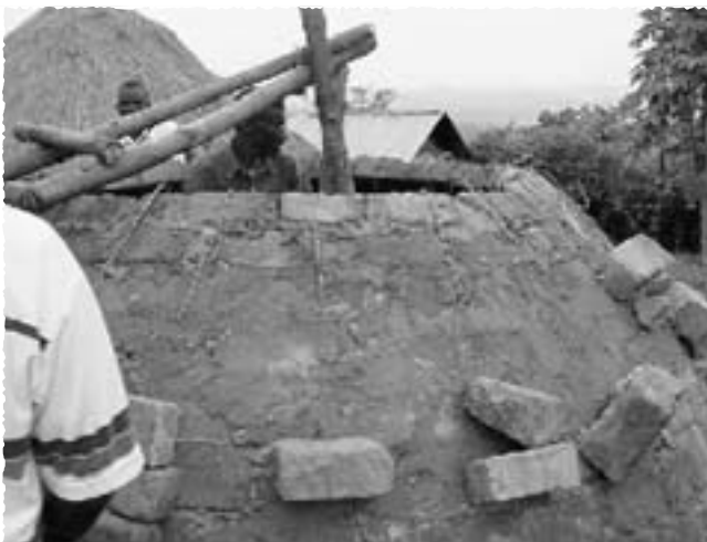
Construction of a spherical tank in Mbarara district, Uganda. Photos: Gedion Shone.
