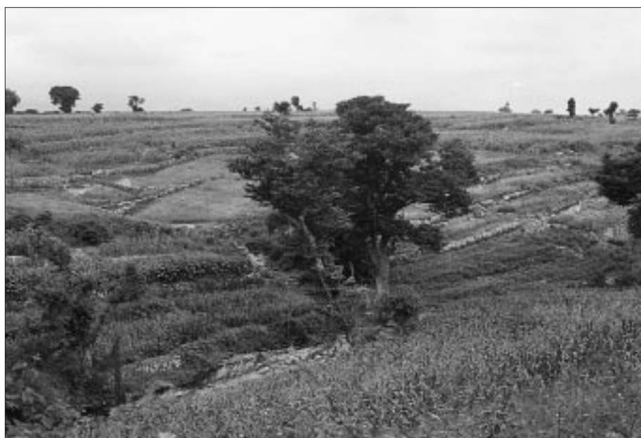
AK Doddi watershed showing stone bunding and bund strengthening with vegetative measures
