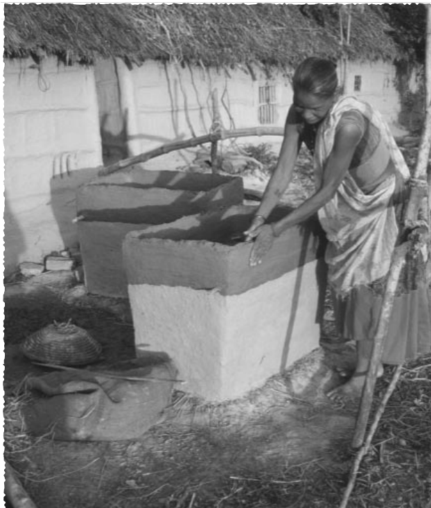
'Dehri-making': Tharu woman of Gobardiha, Deukhuri, building a mud bin for storage of food grain. Photo: Astrid Bjørnsen
