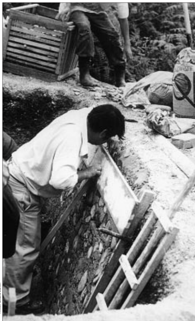
Juan Atz, a farmer experimenter, lines a micro-catchment to prevent seepage.
