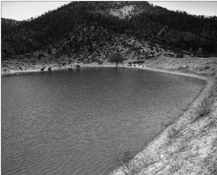
The Johad is a structure bound on three sides by the natural slopes of the hill. The fourth side, a mud wall – usually semi-circular in form – holds back the monsoon run-off.
