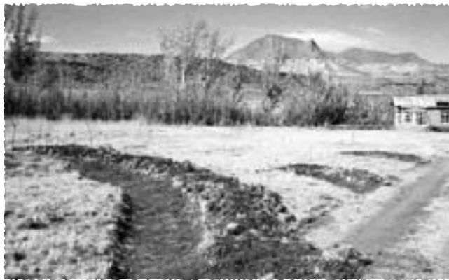
New swale construction. Photo: BBCDC.
