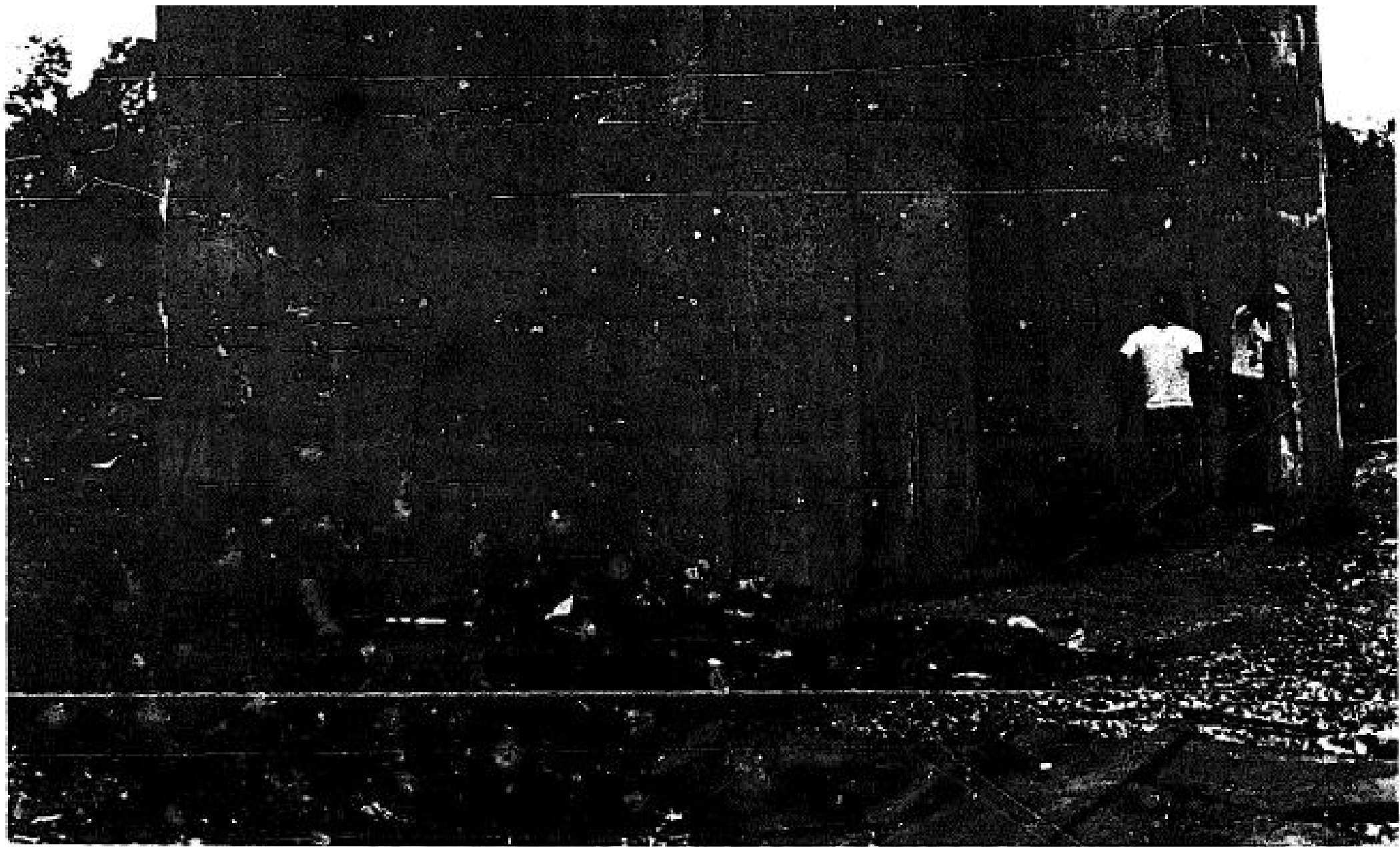
Illustration 2-3: Gas holders for the fourth biogas plant under construction at Maya Farms
