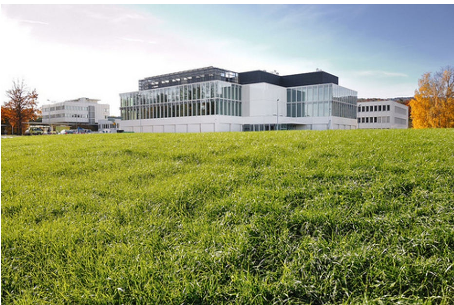
Binnig and Rohrer Nanotechnology Center, Zurich, Switzerland
