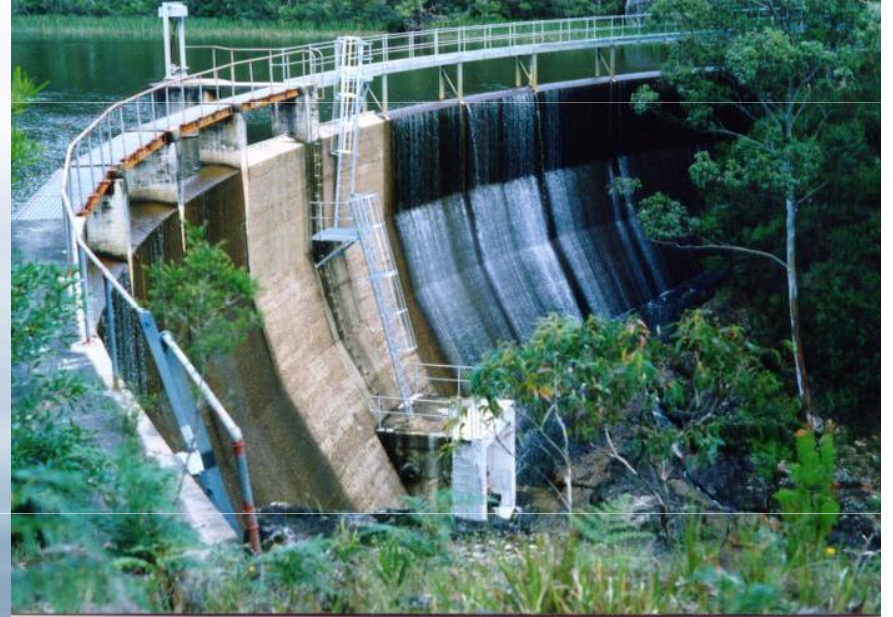
Woodford Creek Dam
