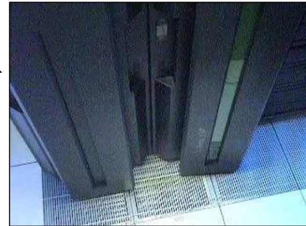
Raised floor tile for behind z10
