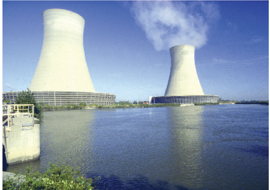
DTE Energy is a 150-year-old company with $9B in revenues and manages $23B in assets. These include Detroit Edison with 2.2 million electric customers, nine fossil units, and the Fermi 2 nuclear power station, generating 11,000 megawatts, as well as MichCon, serving 1.3 million gas customers in Michigan. DTE Energy operates non-regulated businesses in 38 states.
