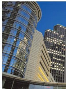
Facility Assets with smart energy, security & emergency systems that alert before failures occur
