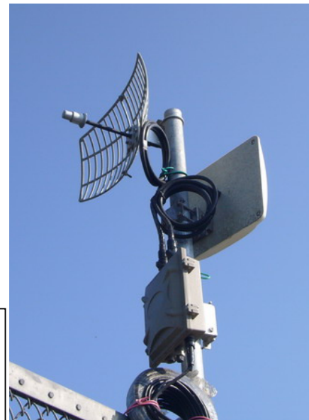
Wrap two layers of insulating tape on connectors to ensure waterproof
