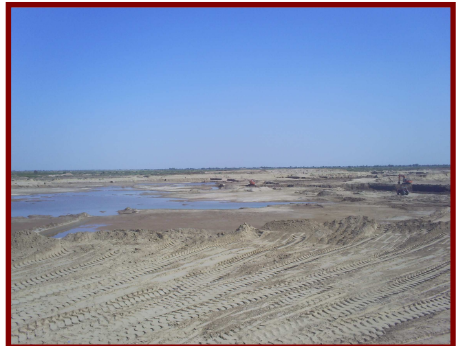
Work under progress
