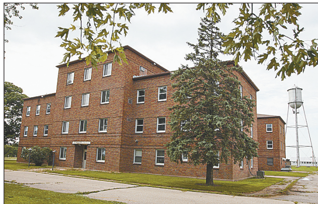
The former Des Moines County Residential facility is located on Washington Road in West Burlington.
