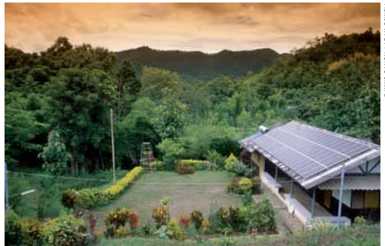
Sankampaeng solenergi station i Chiang Mai, Thailand
