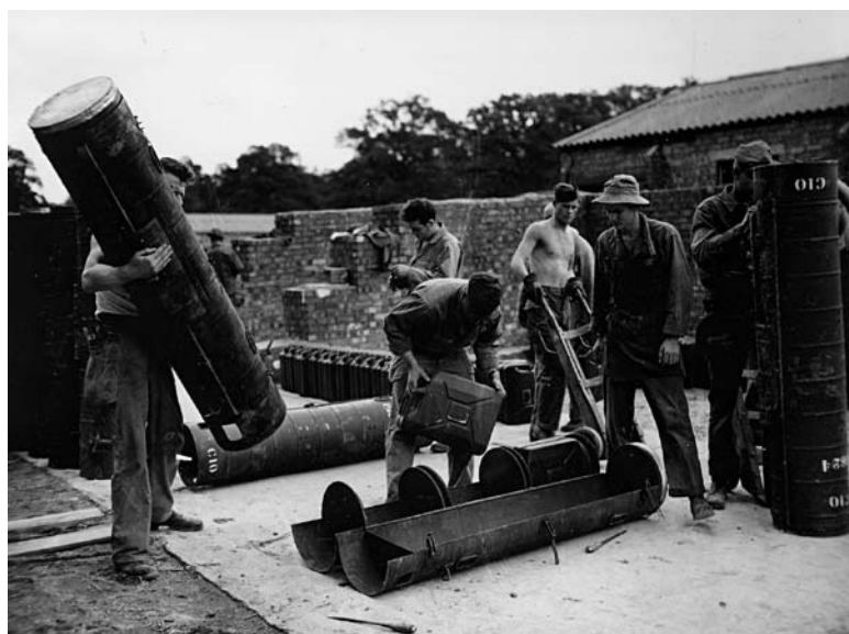
Gasoline being packed in type "C" containers. Notice the brick revetting walls.
