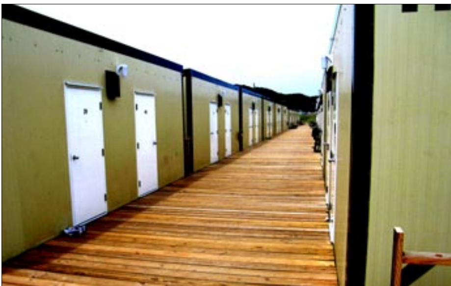
Cuzco Barracks provides individual Troopers with their own living spaces. Cuzco Phase Three, scheduled for completion later this fall, will relieve overcrowding in other housing areas. (Photo by Army Staff Sgt. Paul Meeker)
