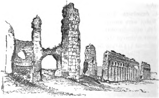
FIG. 193. THE CLAUDIAN AQUEDUCT. (From a photograph)
