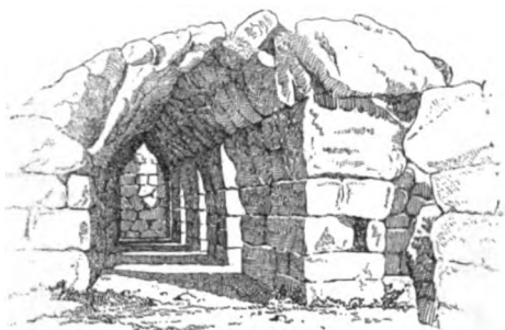
FIG. 74. GALLERY IN THE SOUTH WALL AT TIRYNS
