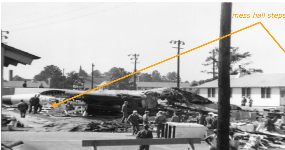
The crash totally destroyed the mess hall but left the adjacent buildings undamaged.
