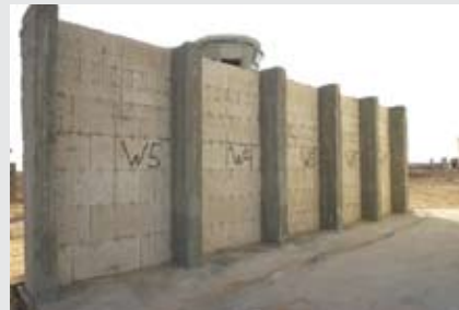
Dynablok™ wall in front of Dynatower
