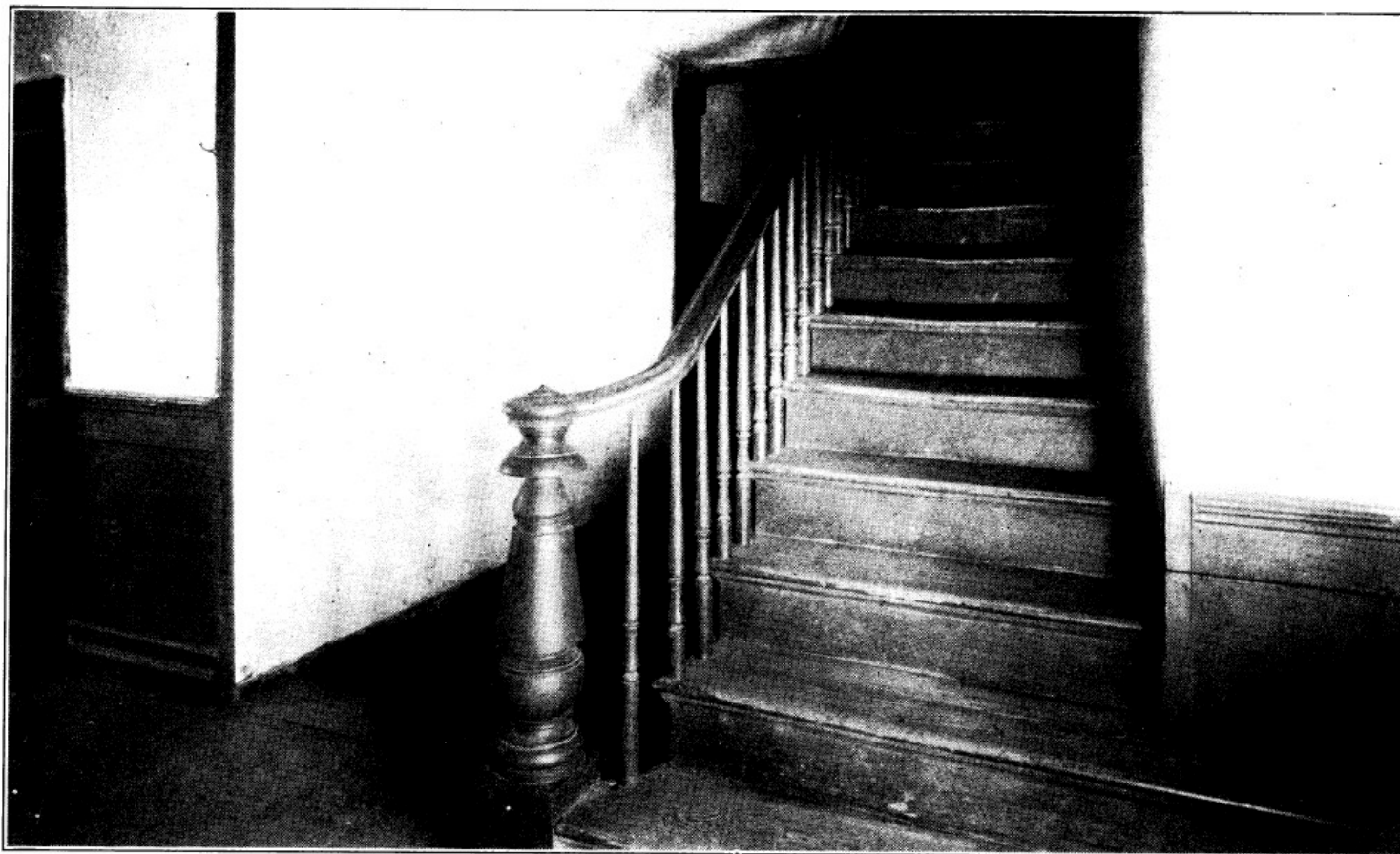
40. Crisscross. Stairway. New Kent County.
