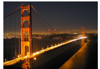
p / The Golden Gate Bridge's roadway is held up by the tension in the vertical cables.
