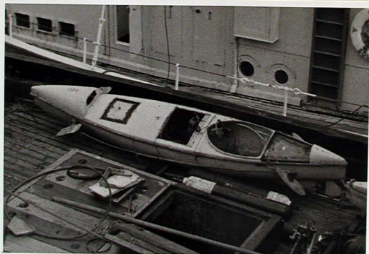
FIG. 2 MOTOR SUBMERSIBLE CANOE SHOWING JURY RIGGED FORE HYDROPLANES AND MODIFIED BOWS
